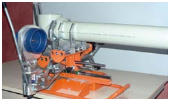
finished weld after cooling period
