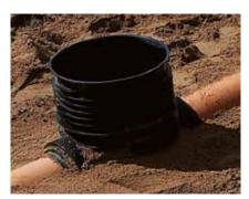
4. In order to immobilize connected sewer node it is recommended to backfill the trench at least 10 cm above the top surface of the sewer pipe. The socket for the shaft pipe should stand out above the backfill.
