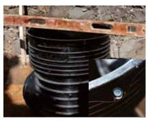
Place the base on the sand bedding and level it out. You may use a level tool placed near the socket connected with the shaft pipe.
