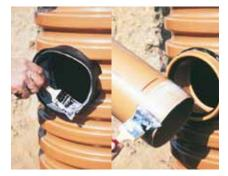
Install a special seal in the opening and lubricate it. Put special "in-situ" socket in the opening.
