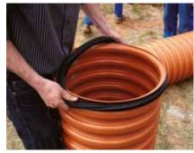
6. Fix the sealing ring delivered with the base on the external side of the pipe between 1<sup>st</sup> and 2<sup>nd</sup> rib. As the sealing ring fixed on the corrugated pipe is profiled, its position must be in line with a drawing on the label.
