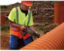
Cut the shaft pipe either manually or mechanically to fit the required height of the chamber. Remember to cut between ribs. Correctly cut pipe should fit (including sealing) in the socket of the shaft pipe.
