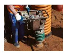
Backfill the trench layer by layer (max. 30 cm) along the entire circumference of the base.
