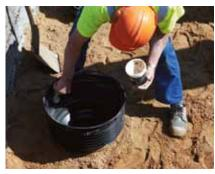
Lubricate the internal side of the socket.
