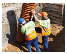
8. Install the pipe with the seal in the base.
