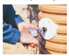
Use special drill crown drill saw to cut an opening in the corrugated pipe. Clean and polish sharp edges of the opening.
