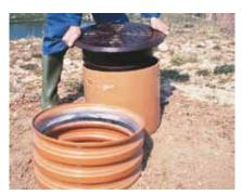
11. If cast-iron covers with telescopic pipe or corrugated pipe are used, fix the sealing ring delivered with the pipes (for corrugated pipes) at the highest groove between the valley of the corrugated pipe. Connect the grating or cover with the telescopic pipe (snap-in-place mechanical connection).
