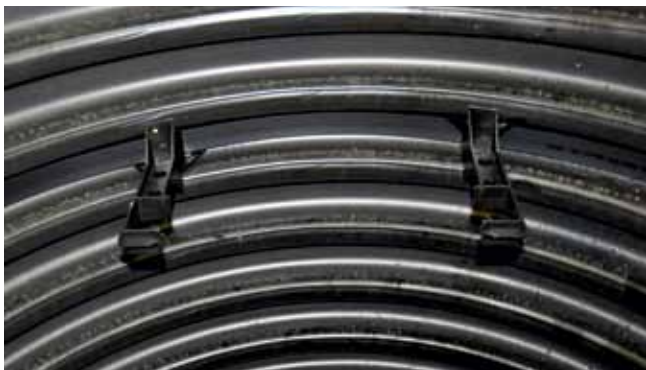
Picture 6. The support strip pre-assembled in the shaft.
