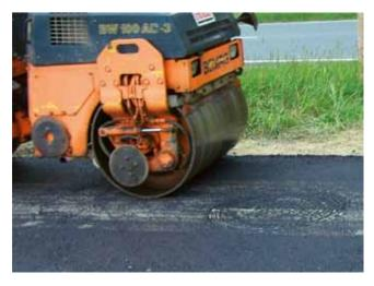
Roll the asphalt layer. When the cover is already installed it should be pressed down first by rolling its middle part without vibrations.
