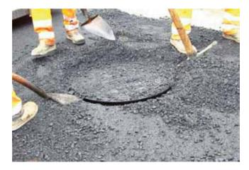
8. Just after finishing this operation move the cover up with telescopic pipe or telescopic adapter by using a pick or a spade.
