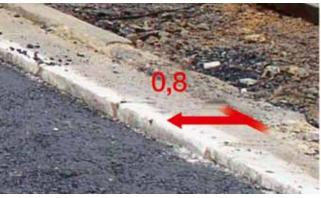
2. . Mark the location of chamber on the shoulder or the curb to allow finding chamber after covering it with asphalt.
