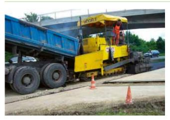
11. Put the asphalt surface by using road finisher.
