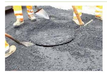
12. When cover with telescopic pipe is used repeat previously made operation – after the road finisher is removed from installation place the cover should be uncovered and moved up (by using e.g. a pick or a spade) to be higher than the non-compacted bituminous layer (min. 20% of the layer thickness).
