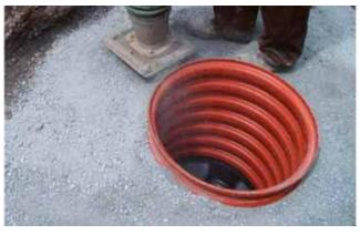
1. Level the upper edge of the chamber about 35 cm under the planned road surface level (on the level the upper freezeproof layer). Compact thoroughly the soil around the chamber beginning from its bottom part. The soil shall be compacted layer by layer (max 30 cm) according to the chamber installation guide. Protect backfilling against washing out in line with PN-EN 1610 and PN-ENV 1046.
